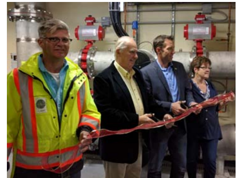
Delegates cutting the ribbon in front of the new UV system
