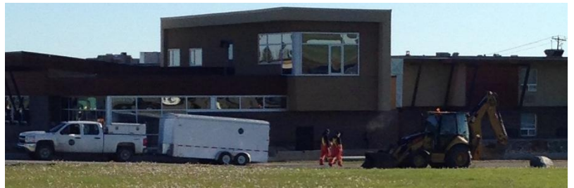
Figure 3: Water service repair at Heritage Inn.
