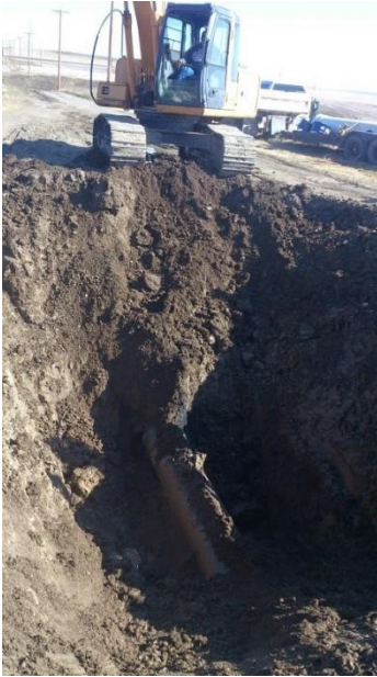
Figure 5: Force Main Repair
