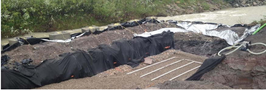
Figure 6: Raw Water Intake Project
