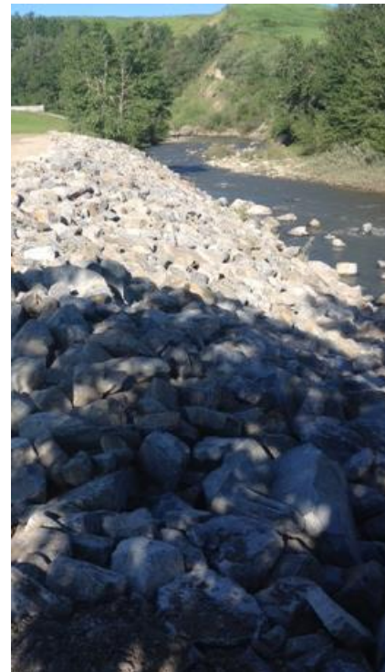
Figure 7: Completed creek bank at water intake site
