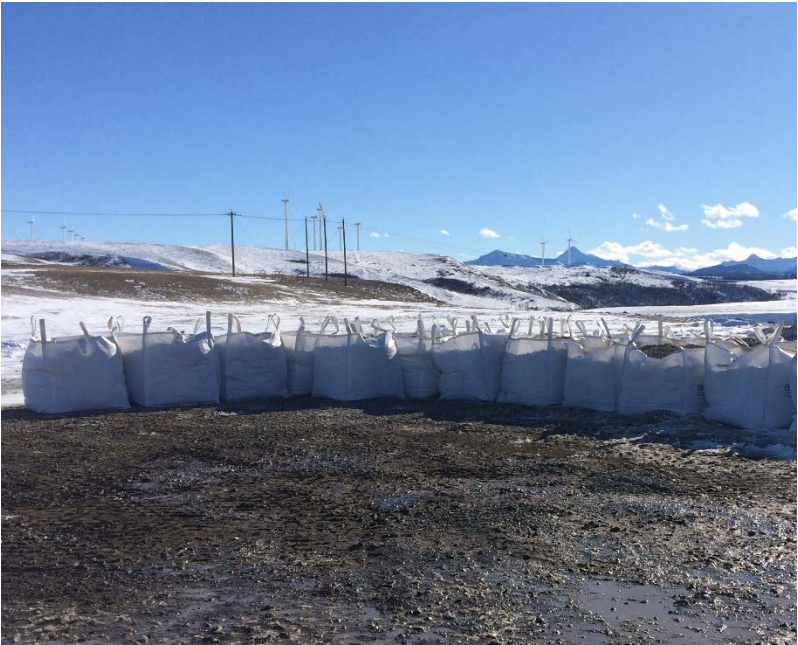
Sand bags used for damming Castle River
