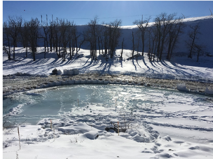
Castle Raw Water Intake
