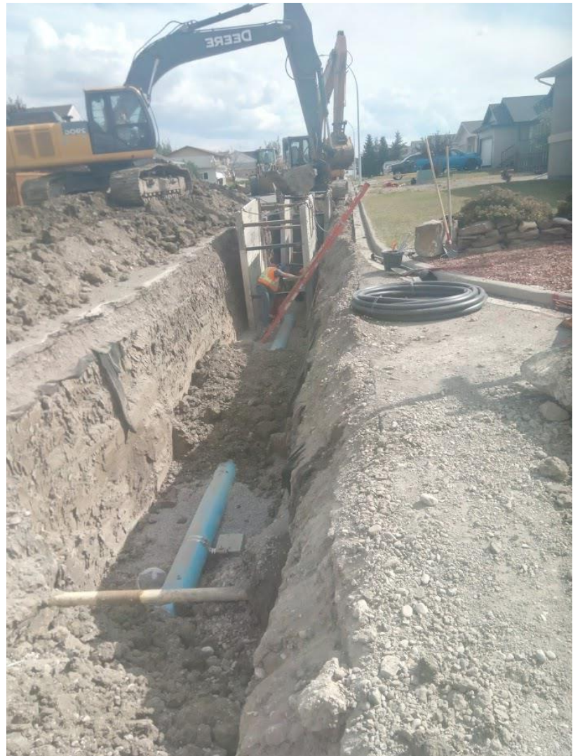
Thistle Crescent water line upgrades
