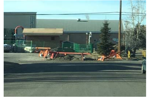
Spray Park Construction
