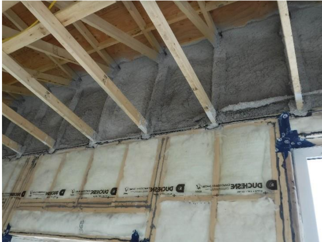
Spray Foam and Insulation Detail
