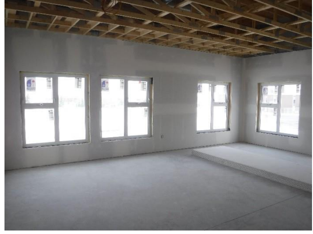
Interior Drywall, Mud and Tape
