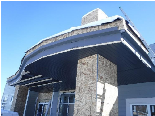
Soffit Under Entrance
