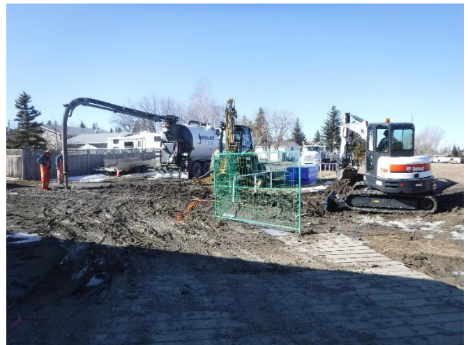
Alta Gas and Town Valve Relocation
