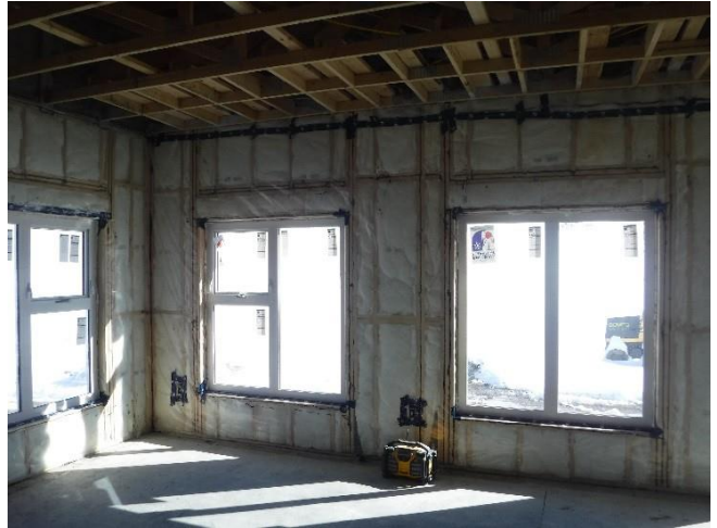
Insulation and Vapor Barrier
