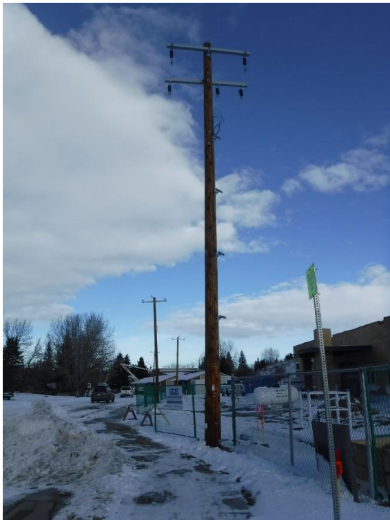
Power Pole Installed for Fortis
