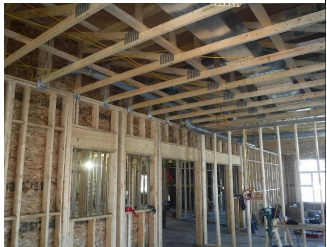
Roof Drain and HVAC Rough-In
