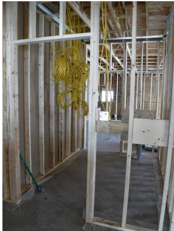
Interior Framing and Electrical
