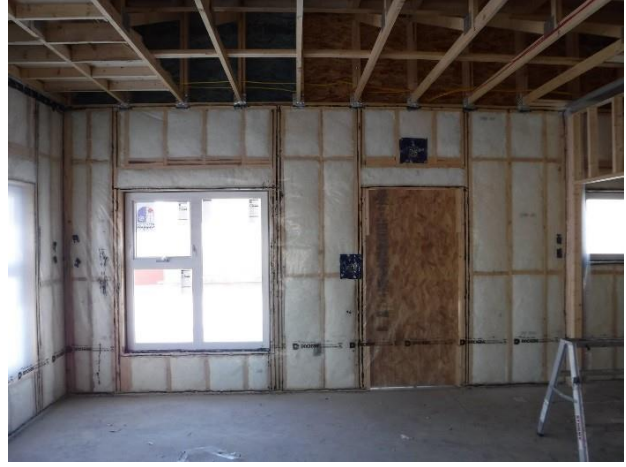
Interior Insulation and Vapor Barrier
