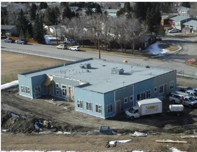
Final Roof Layer Installed
