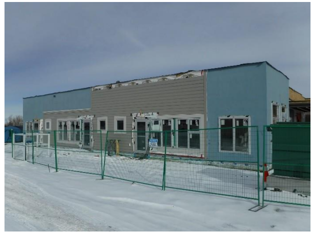
Exterior West Facing Wall
