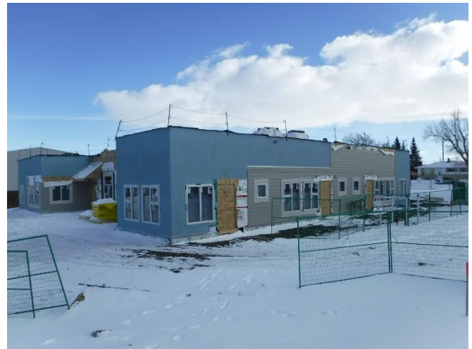
Exterior West Facing Wall
