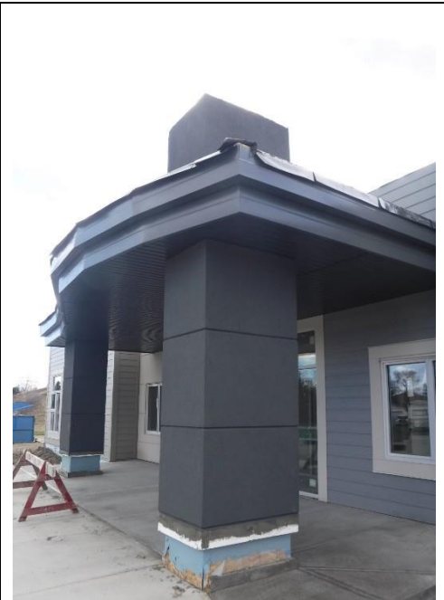
Stucco for Entrance Pillars
