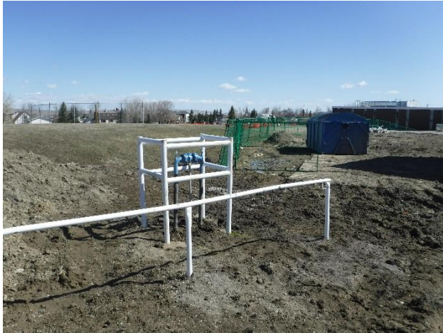
Bollard Cage Installed by Alta Gas
