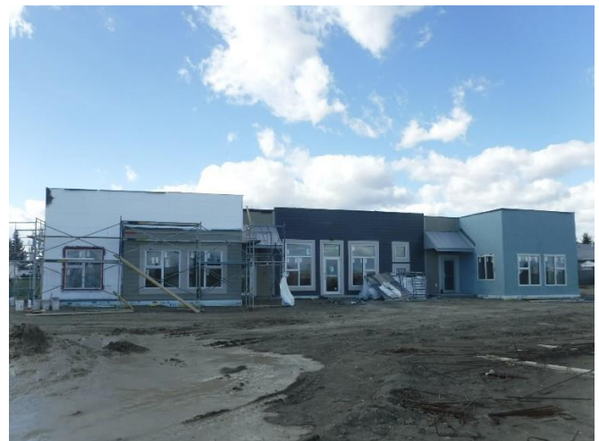
Rear of Building Stucco Preparation
