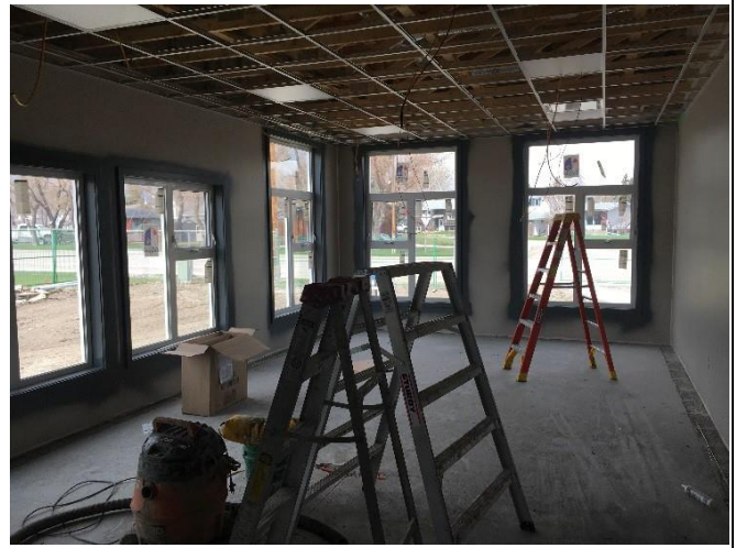
Interior Painting Underway
