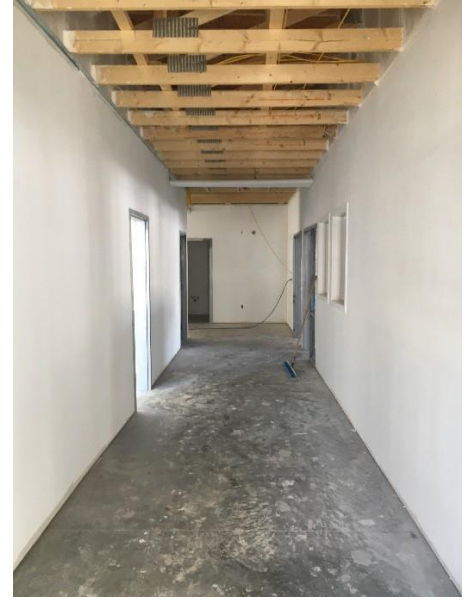
Dry walling Completed
