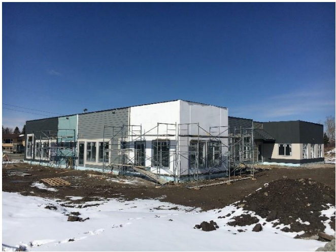
South-West Corner Stucco Preparation
